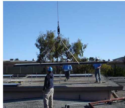
Dismounting and flying out one of seven roof-installed solar panels.
